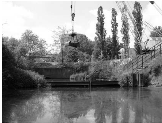
Fig. 3. Sampling point of Sample 1 – Levee
